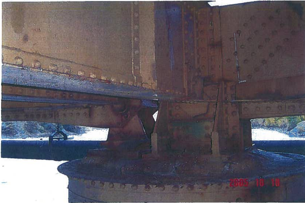
Photo 11: Typical Condition of the Bearings (Pier 1 downstream side shown)
